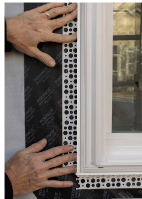
Press it into Place for a Tight Weatherproof Seal without the Need for Caulk or Any Additional Attachments. Corners Can be Caulked if Needed
